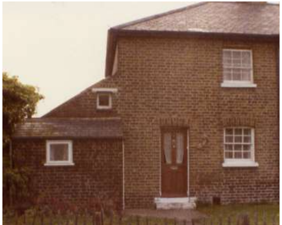
Meadow Lane side of No.1 Brocas Terrace showing lean-to sculleriy and outside toilet and rear entrance
