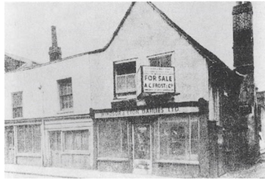
107/108 Windsor & Eton Dairy prior to demolition
